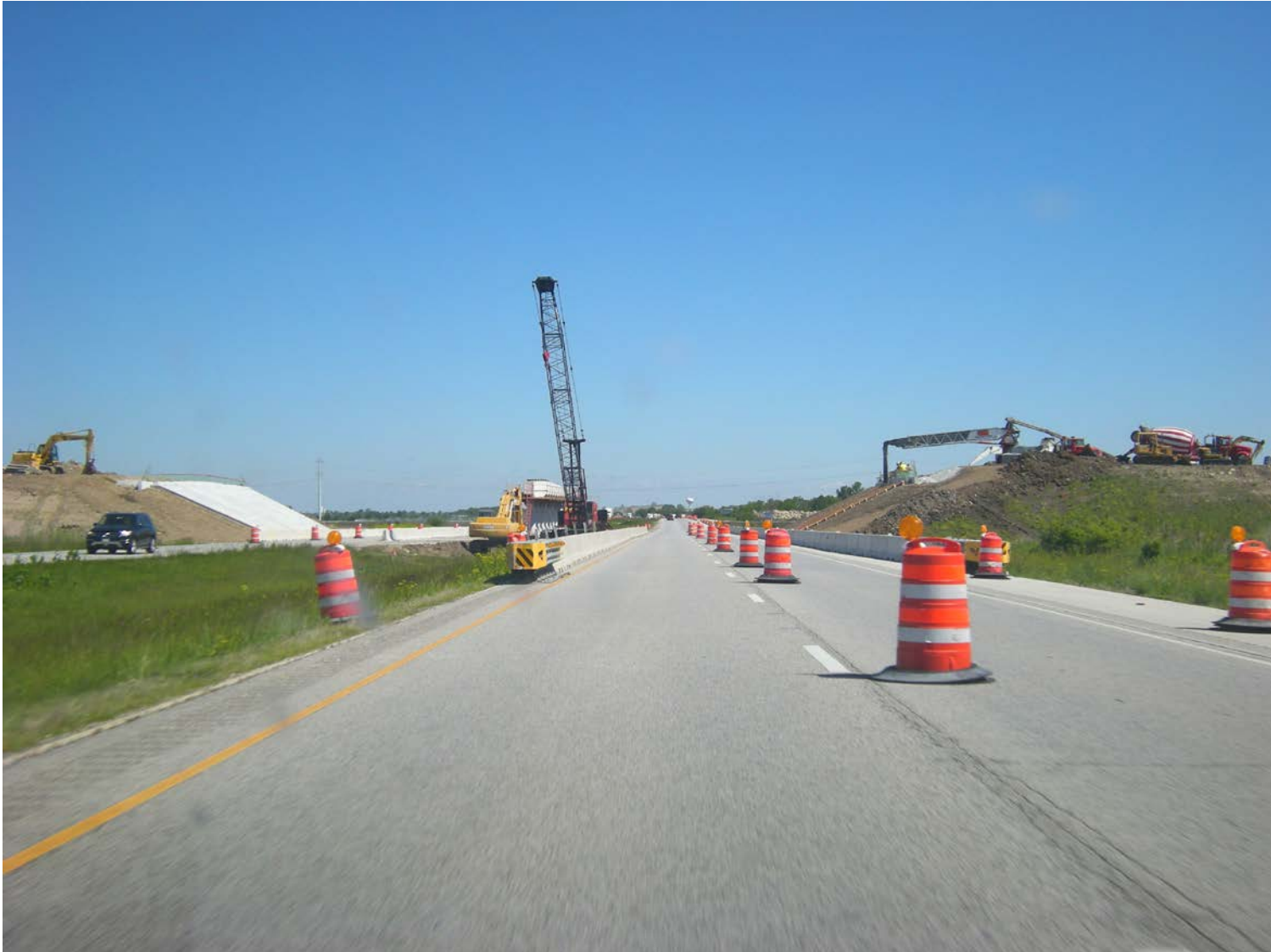
Picture A: I-57 & Bourbonnais Parkway Interchange
