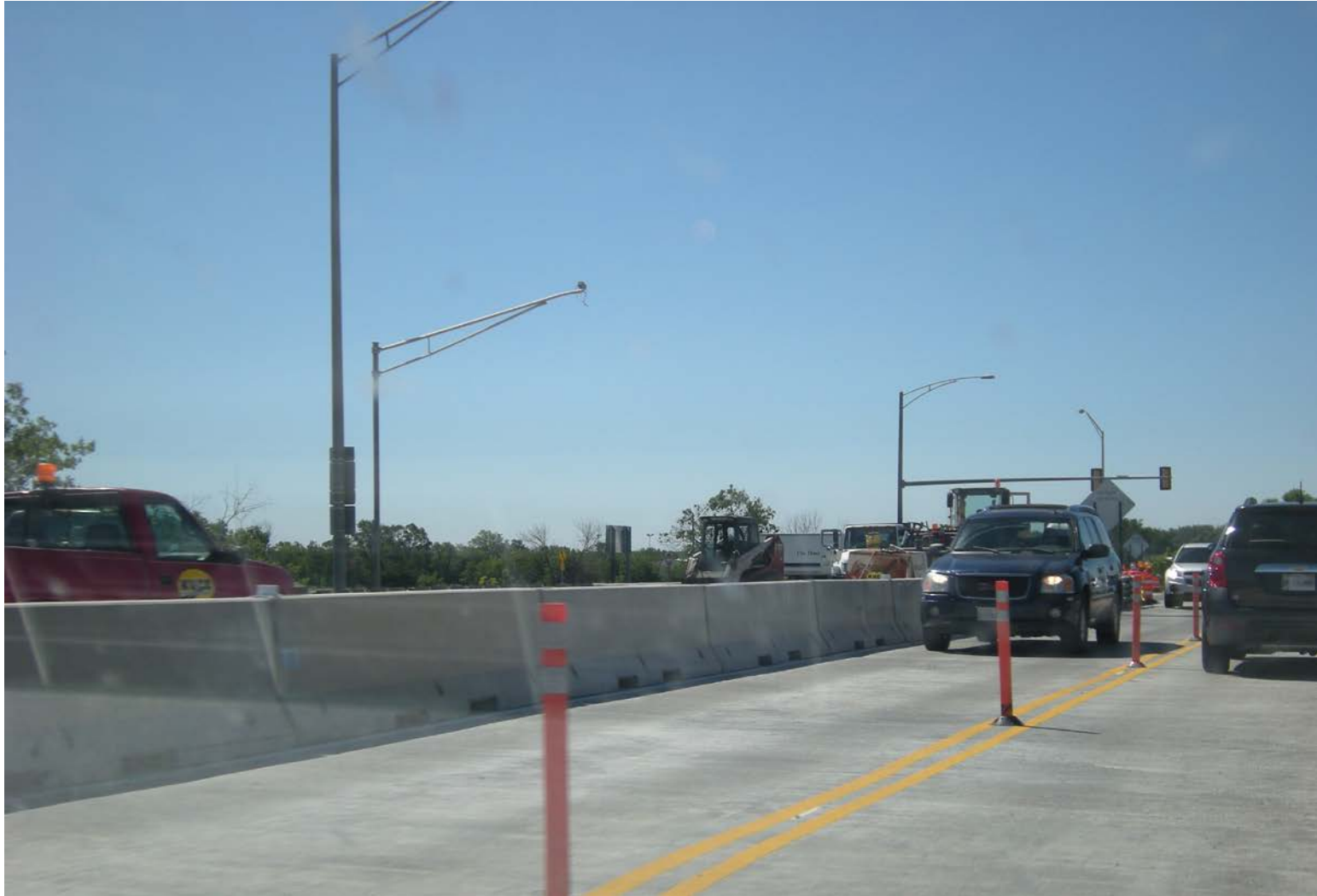
Picture B: Resurfacing of U.S. 45/52 at I-57
