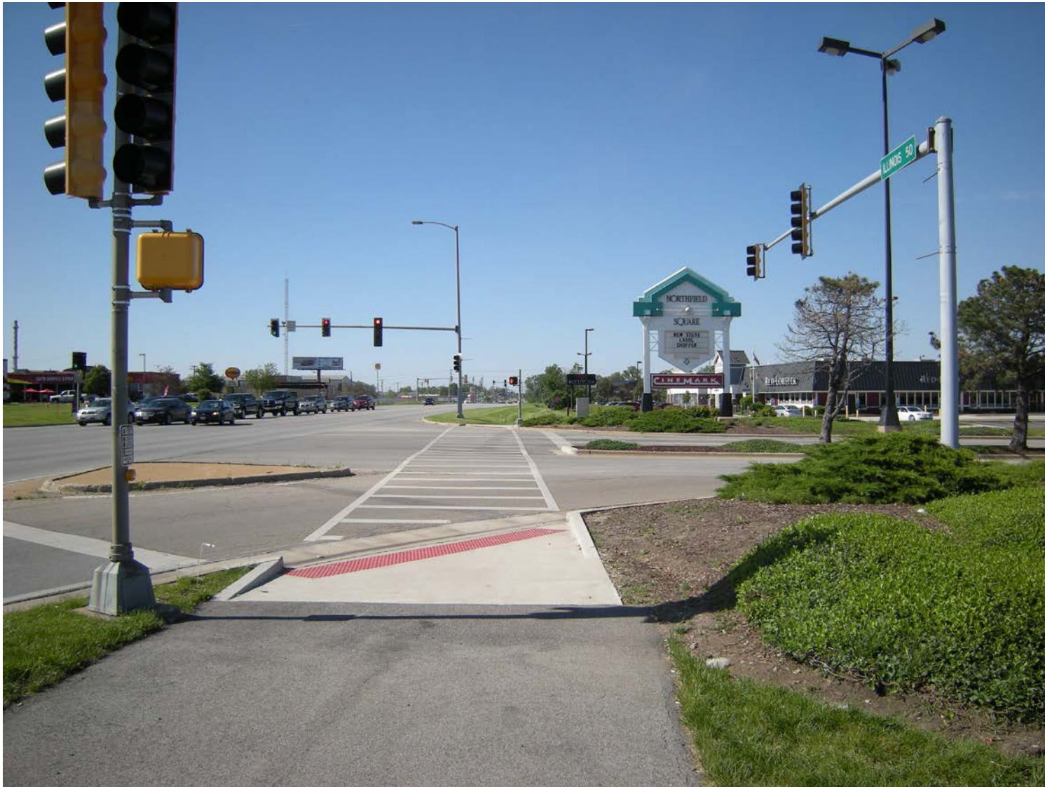
Picture B: Completed Multi-Use Path at IL-50 and Ken Hayes Dr
