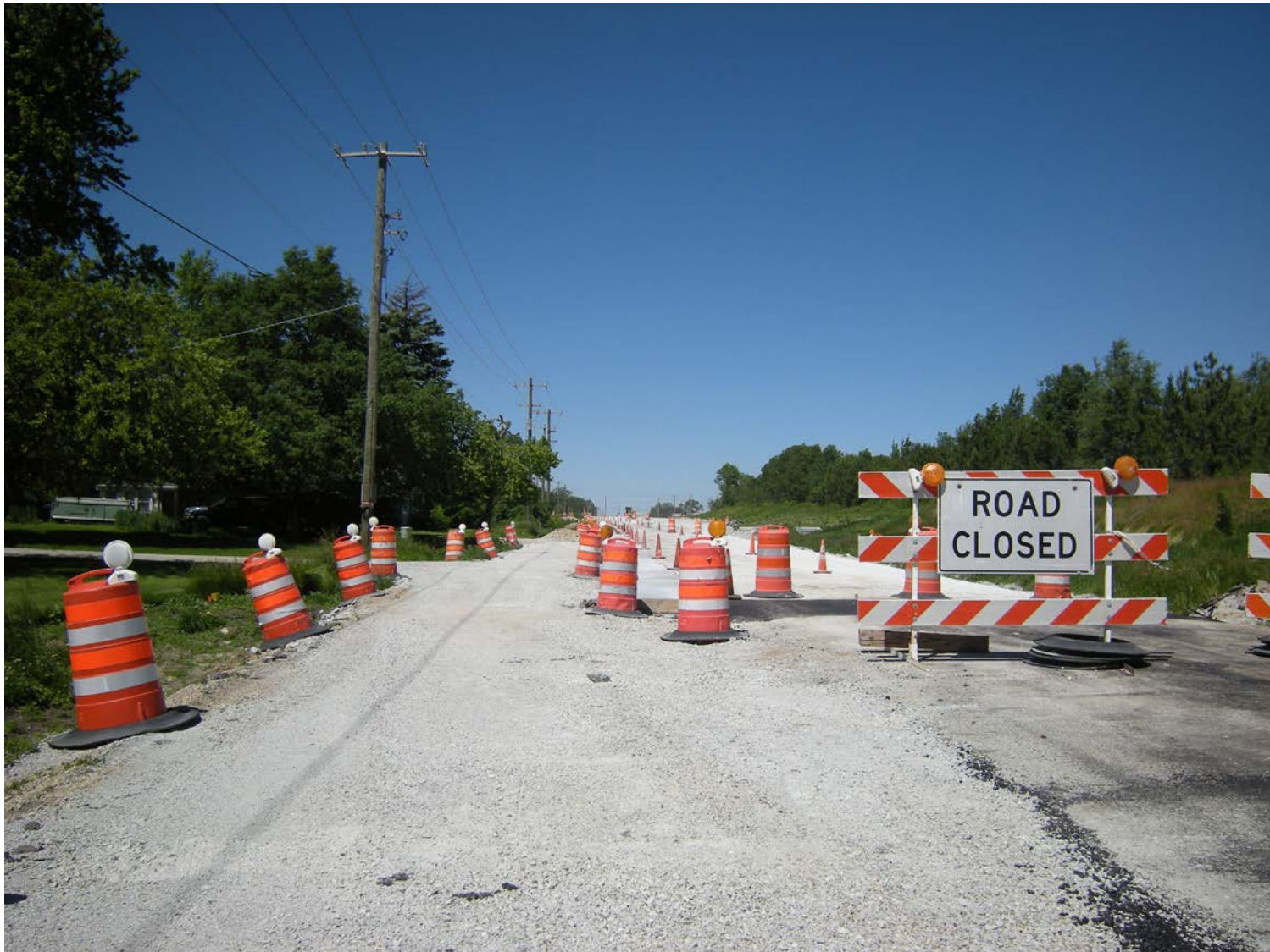
Picture B: 6000N Road west of IL-50
