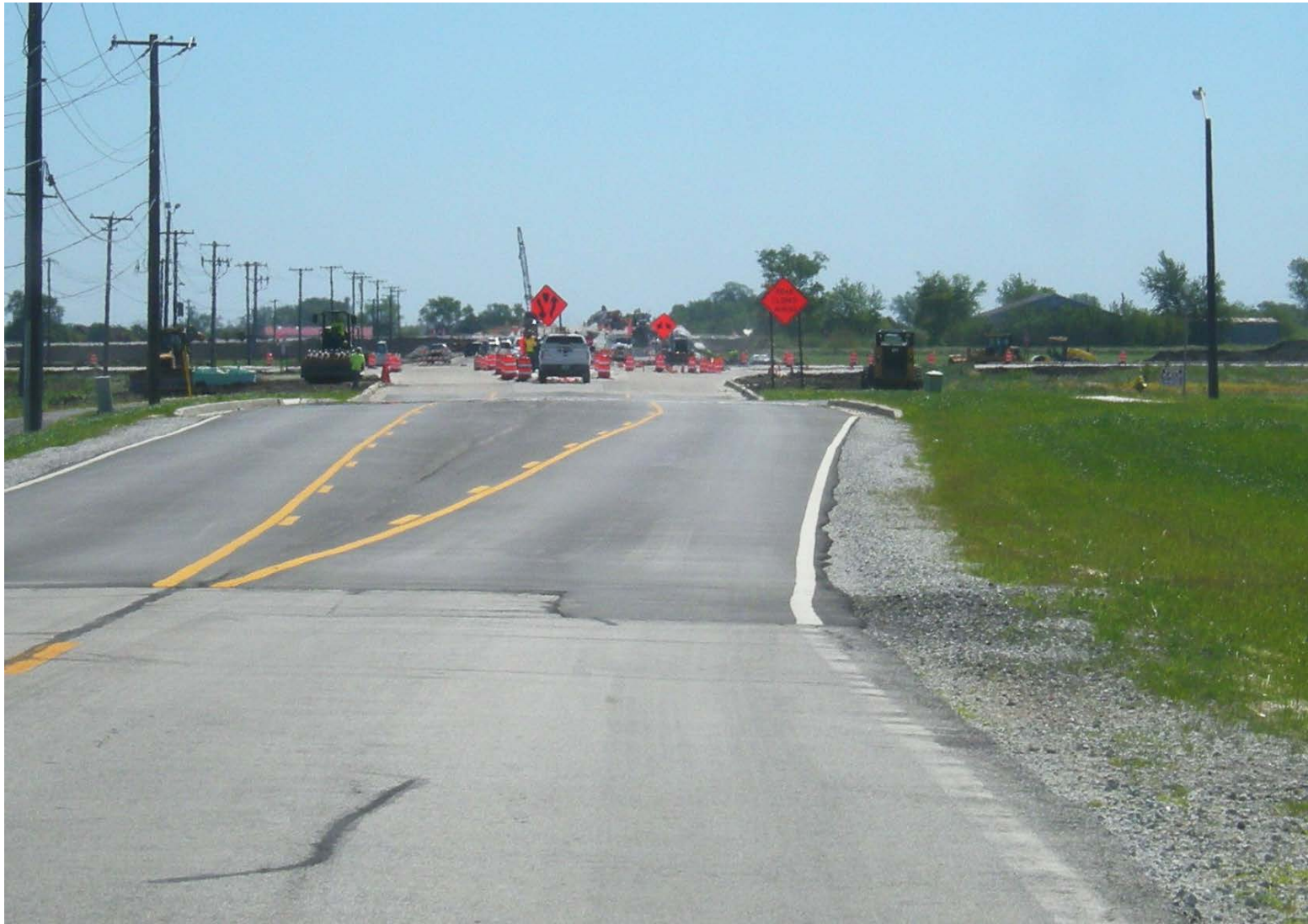
Picture A: Bourbonnais Parkway Widening Project
