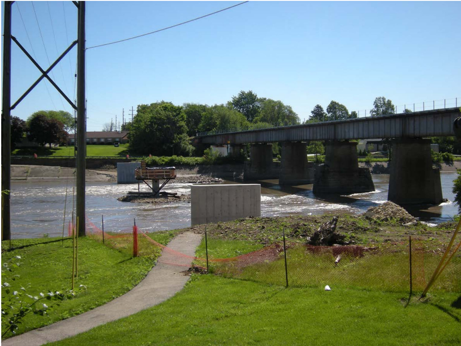
Picture A: Multi-Use Path Construction Over the Kankakee River
