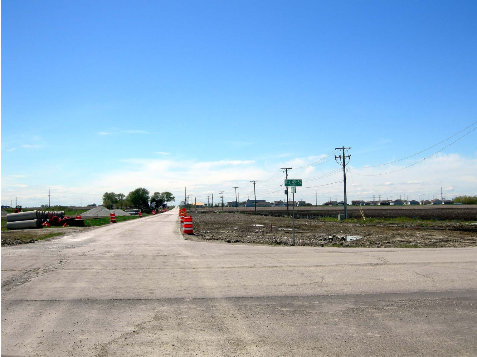
Picture A: Bourbonnais Parkway Widening Project (May 2, 2016)
