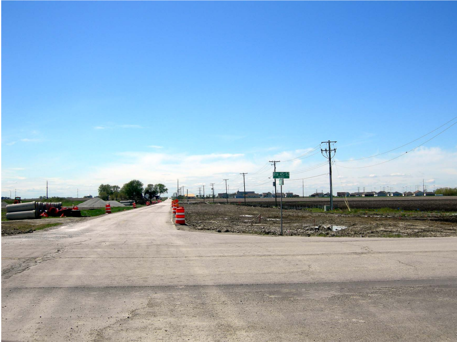
Picture A: Bourbonnais Parkway Widening Project (May 2, 2016)
