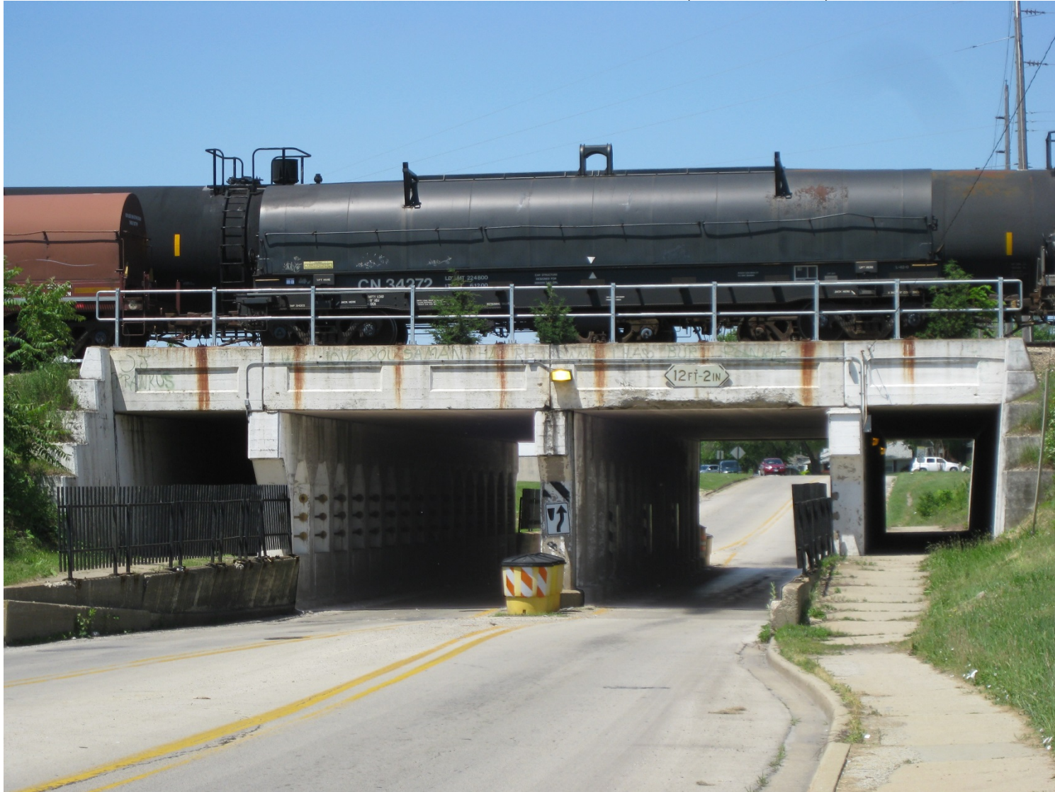
Picture A: Brookmont Boulevard Viaduct (June 2, 2015)
