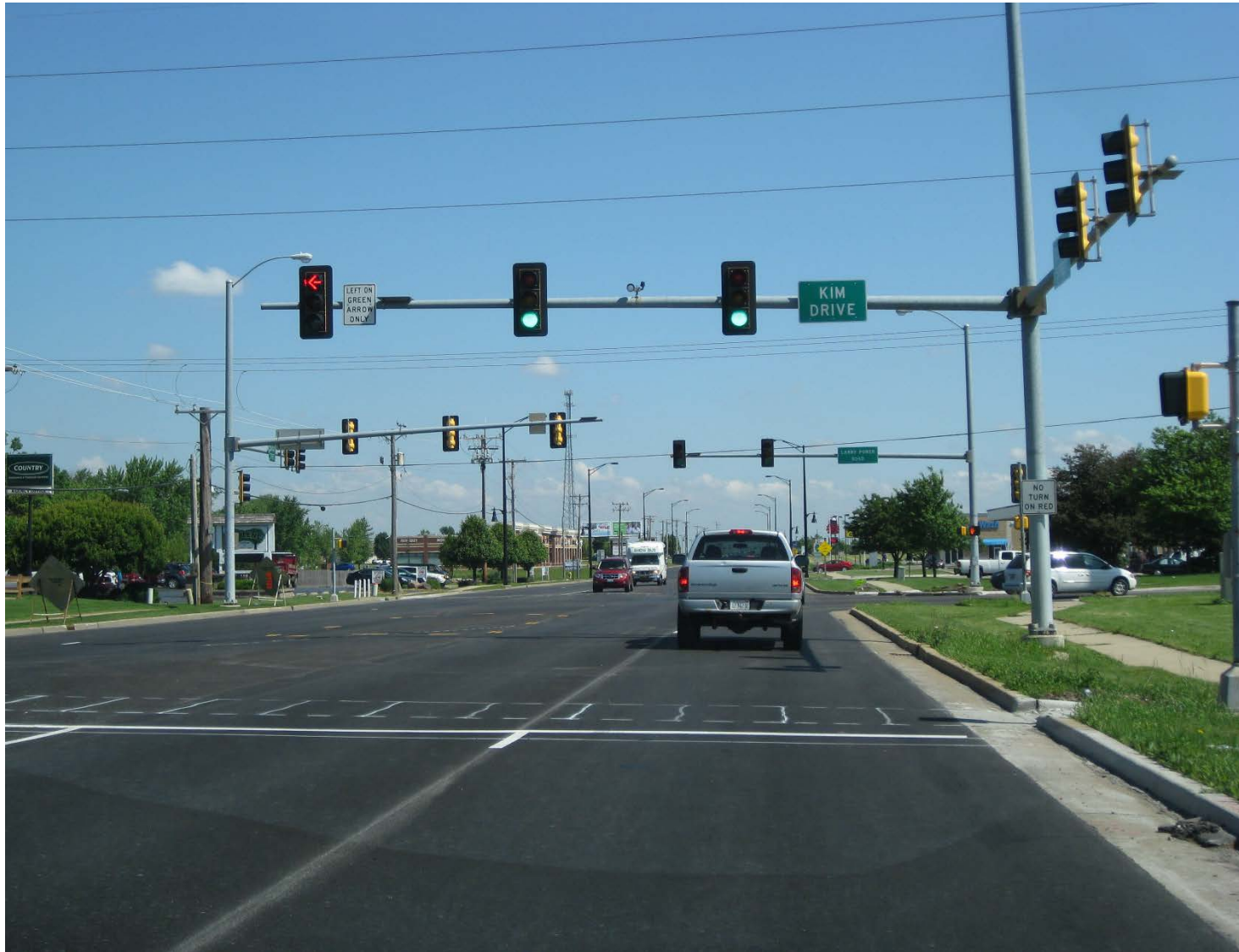
Picture B: Resurfacing U.S. 45/52 at Larry Power Road (June 2, 2015)
