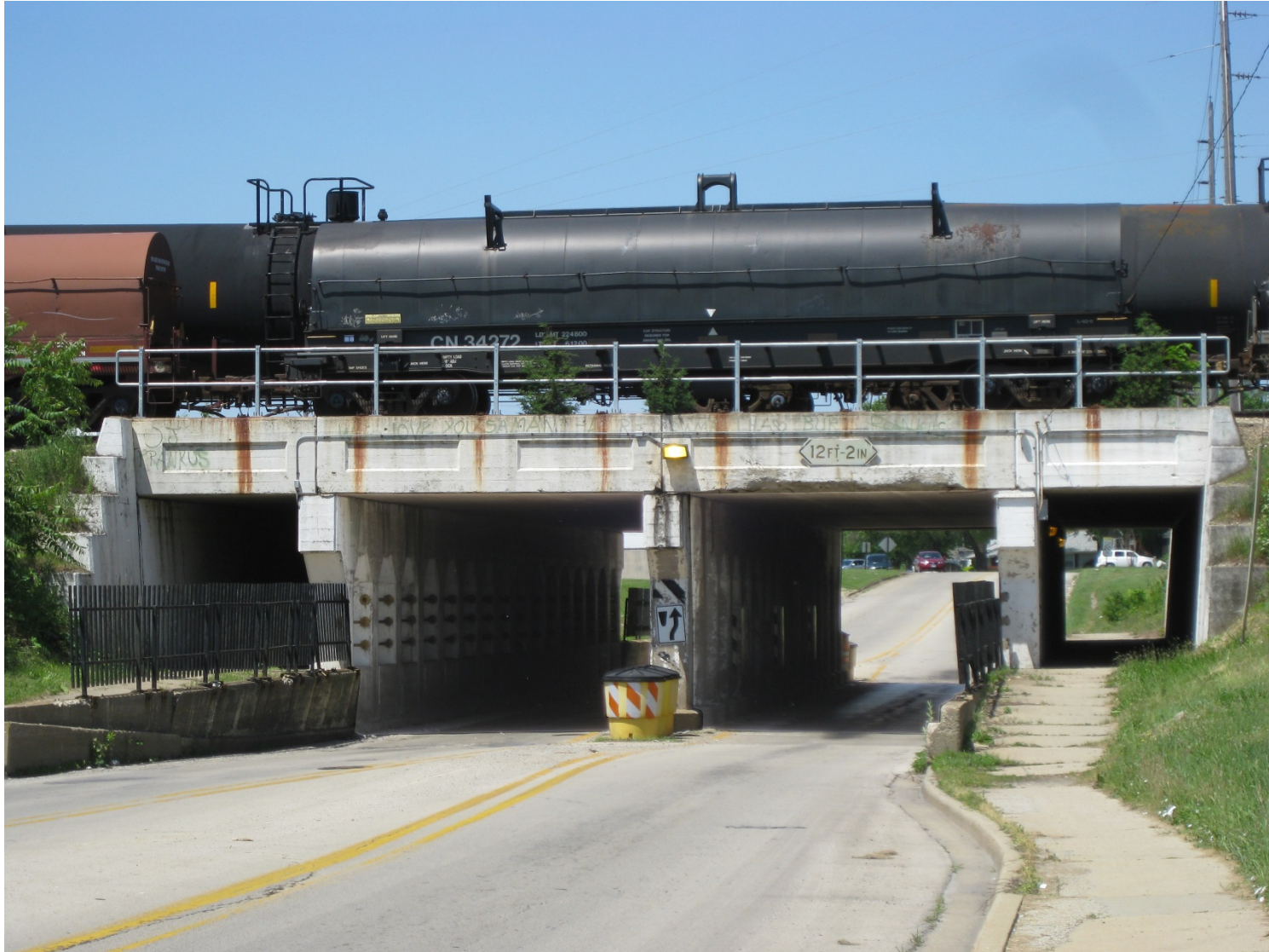
Picture A: Brookmont Boulevard Viaduct (June 2, 2015)
