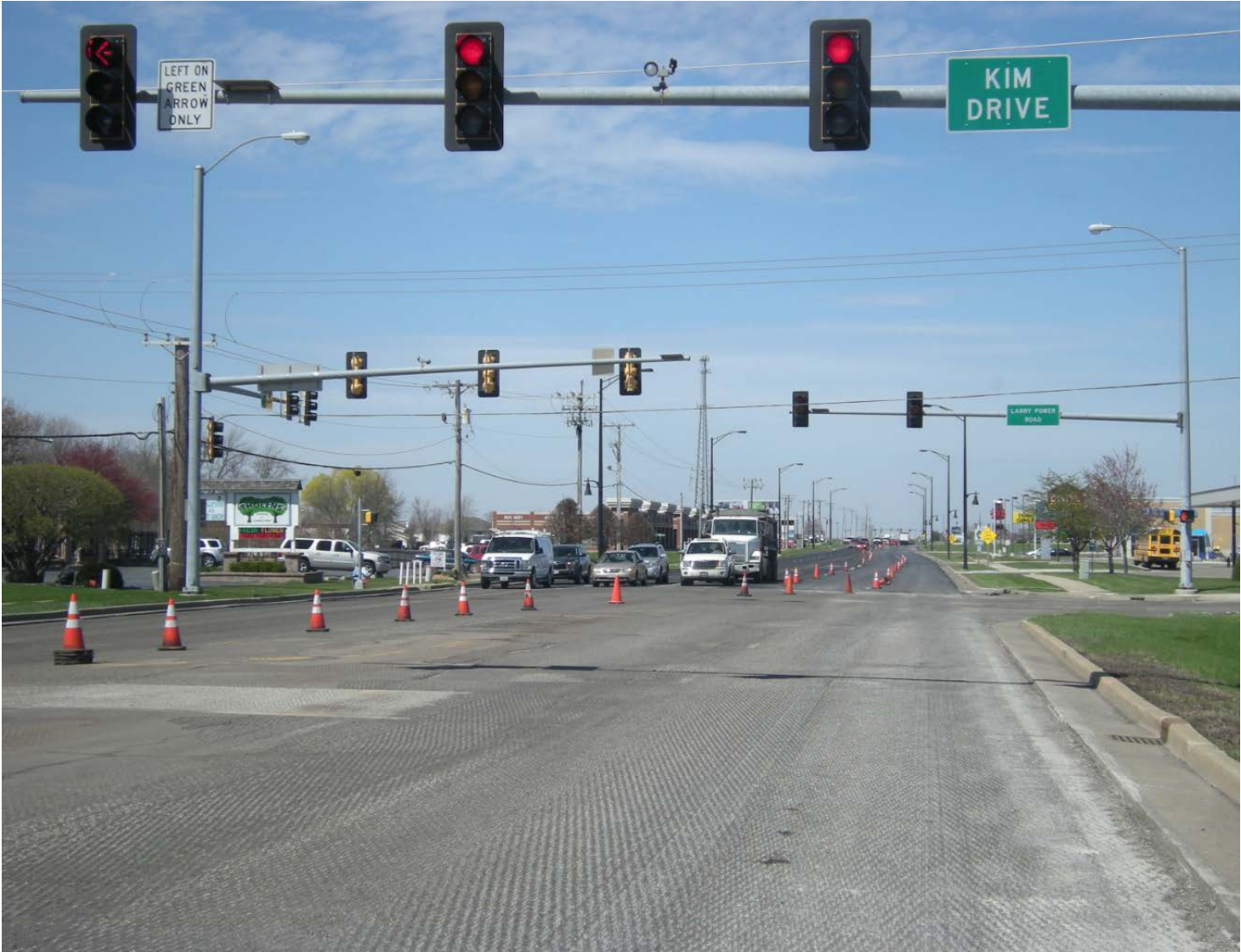
Picture A: Resurfacing U.S. 45/52 at Larry Power Road (April 15, 2015)
