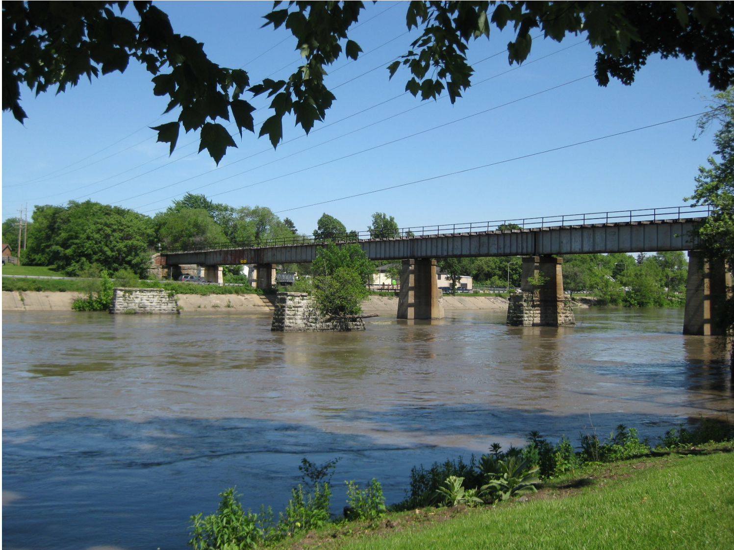
Picture A: Riverfront Trail Phase 2B Bridge Location
