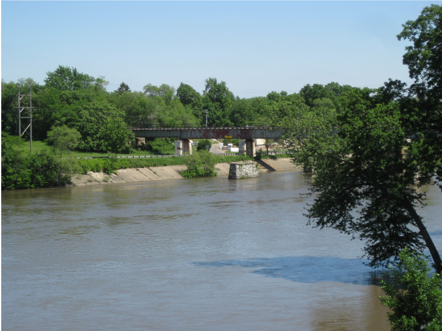
Picture B: Riverfront Trail Phase 2B Bridge Location
