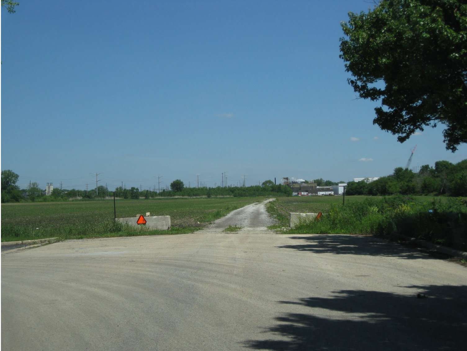
Picture B: Industrial Drive Expansion Project (June 2, 2015)
