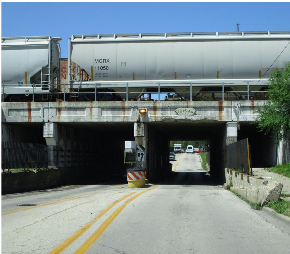
Brookmont Boulevard Viaduct in Kankakee
