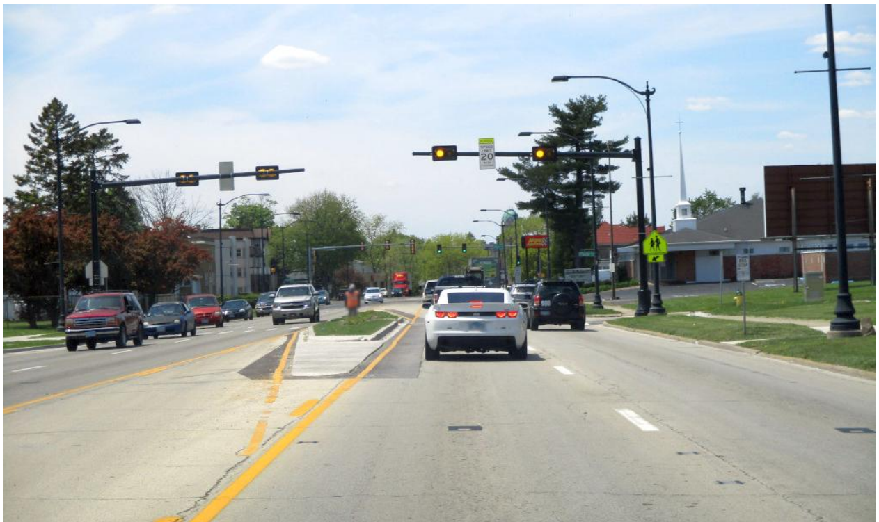
New pedestrian improvements on IL-17 (Court St).
