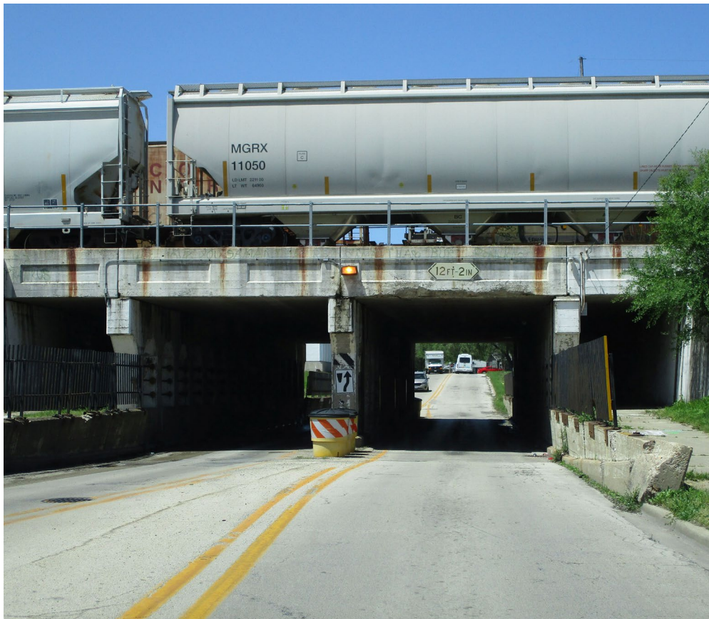
Brookmont Boulevard Viaduct in Kankakee
