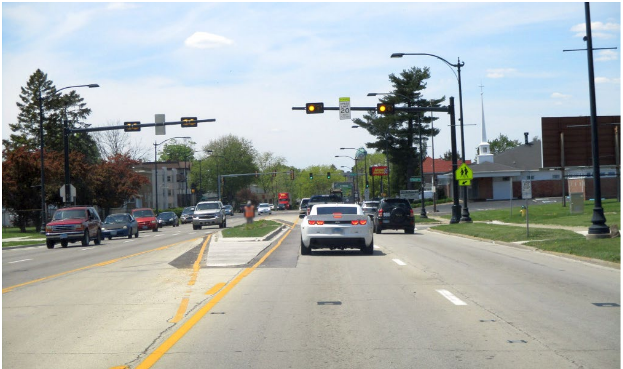
New pedestrian improvements on IL-17 (Court St).
