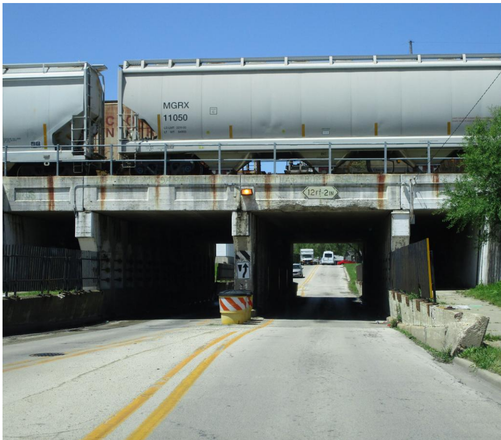
Brookmont Boulevard Viaduct in Kankakee
