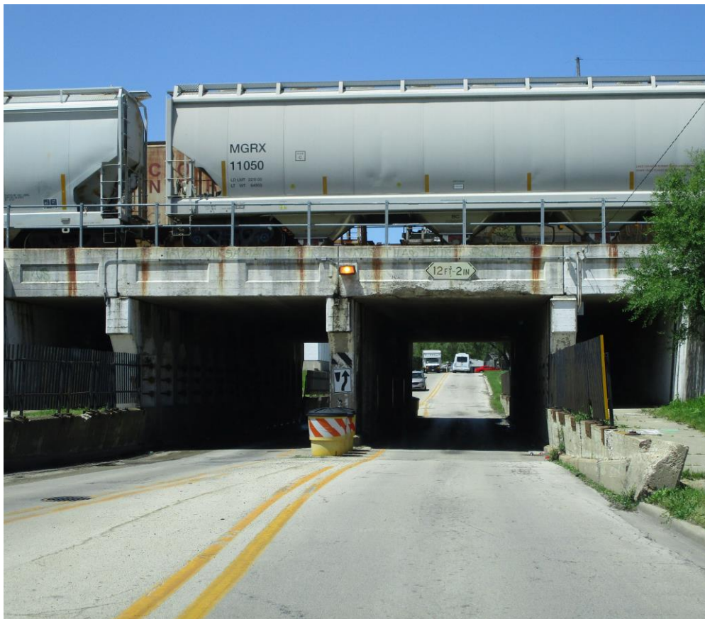
Brookmont Boulevard Viaduct in Kankakee
