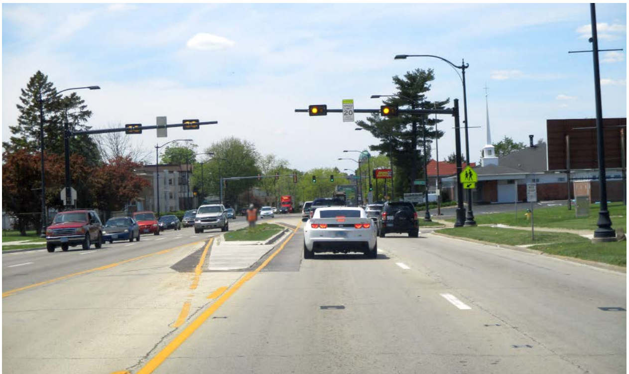
New pedestrian improvements on IL-17 (Court St).
