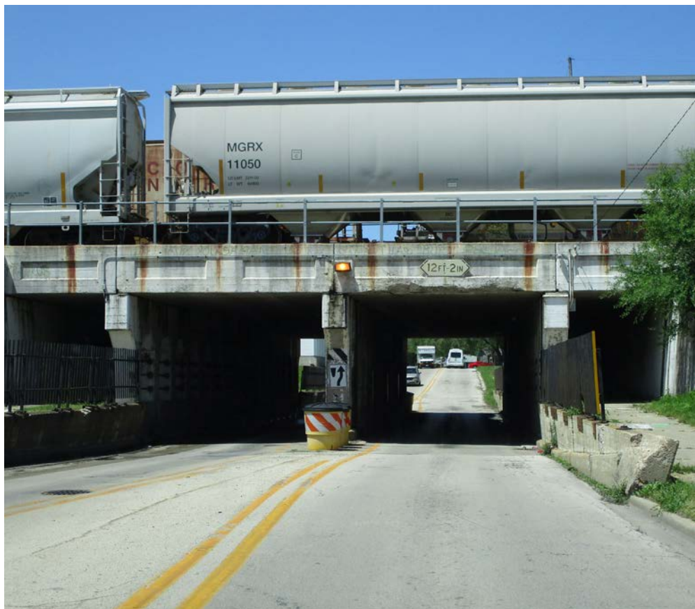
Brookmont Boulevard Viaduct in Kankakee
