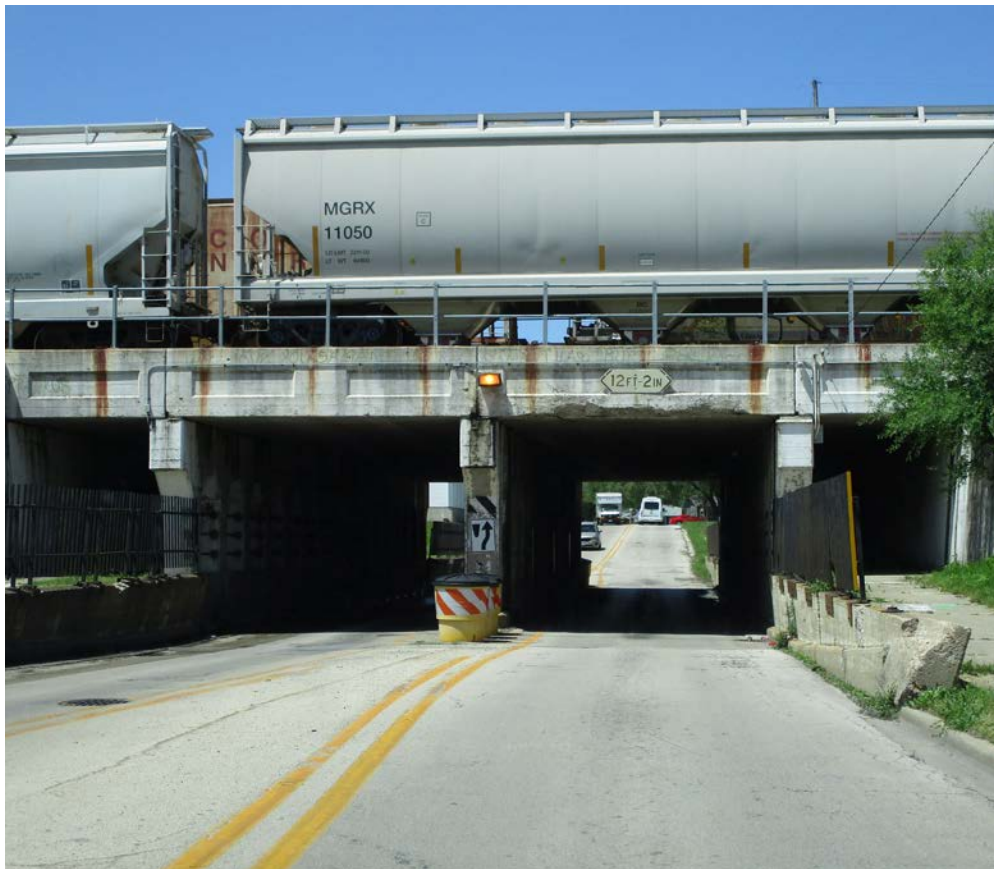
Brookmont Boulevard Viaduct in Kankakee
