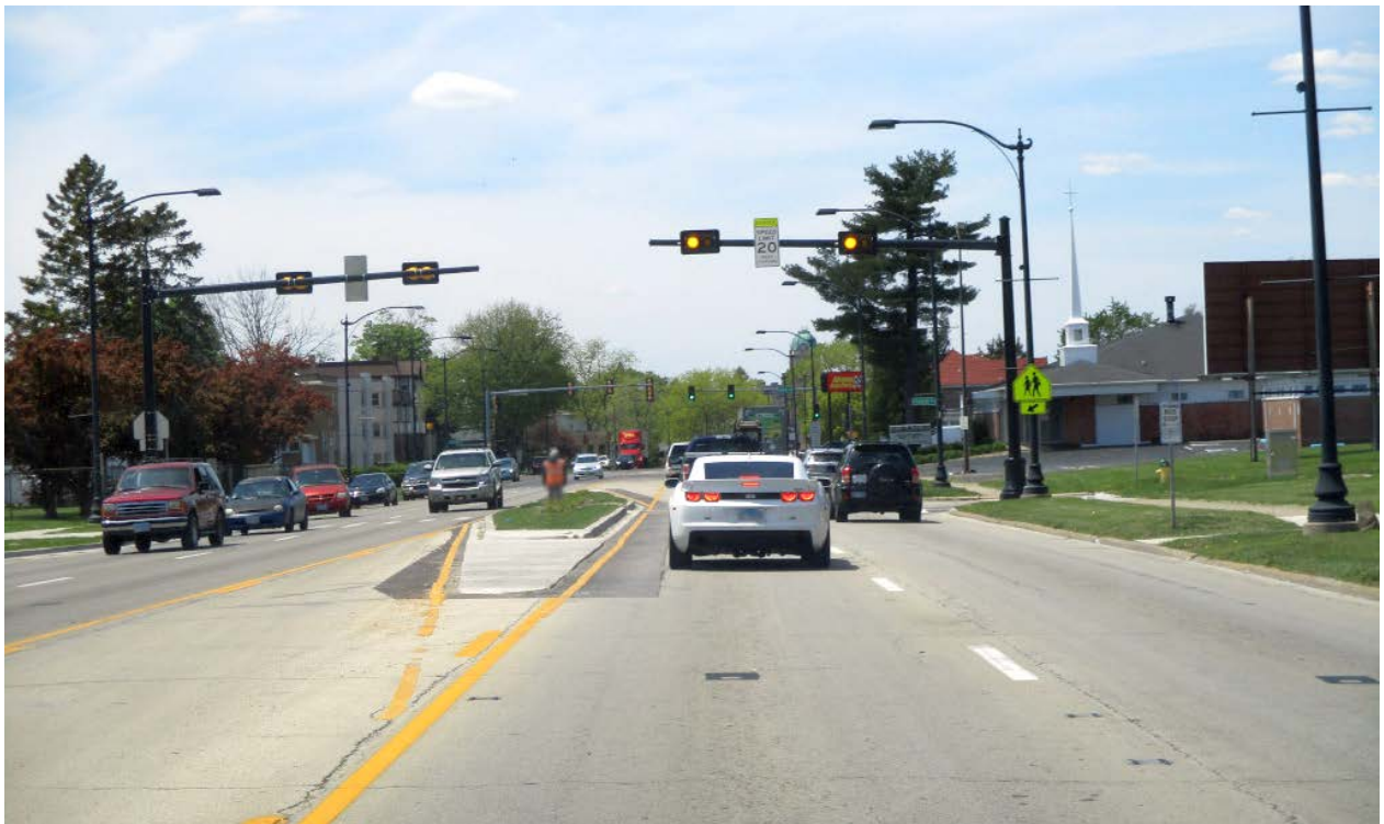
New pedestrian improvements on IL-17 (Court St).
