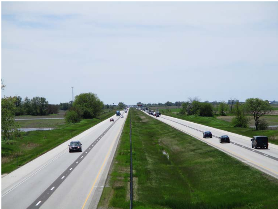
I-57 Looking South from 12000N Rd
