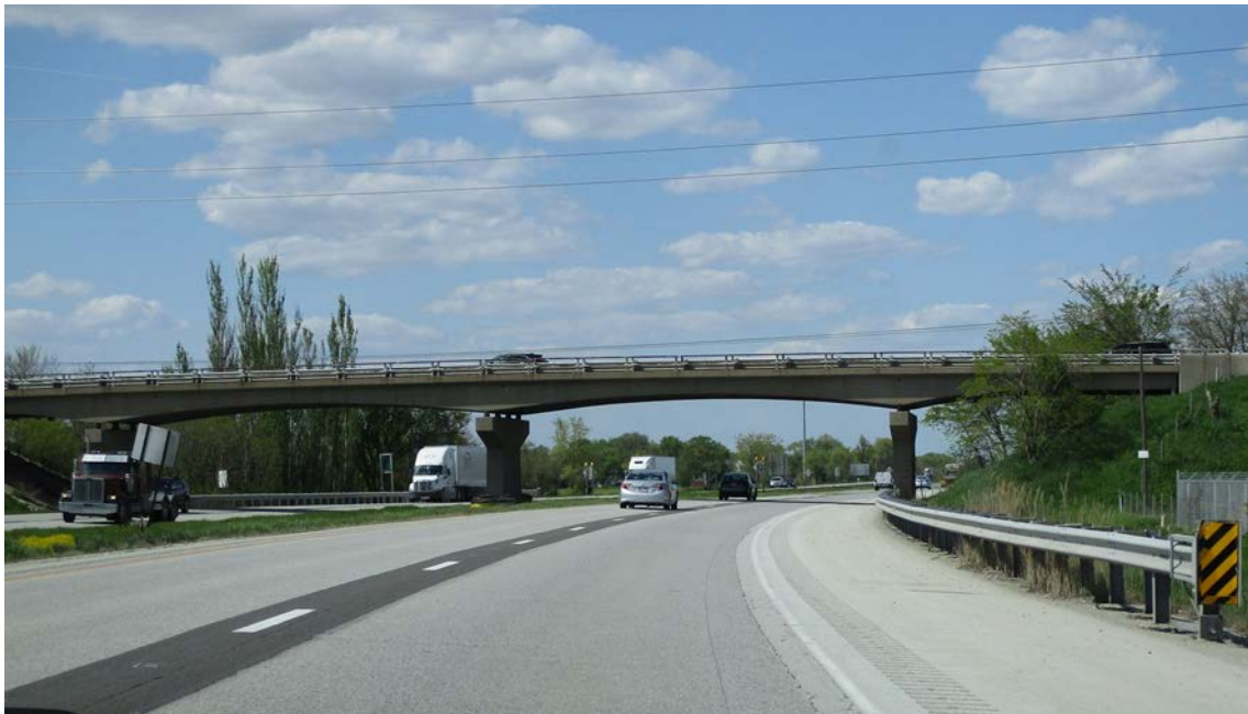
I-57 at Larry Power (4000N) Road
