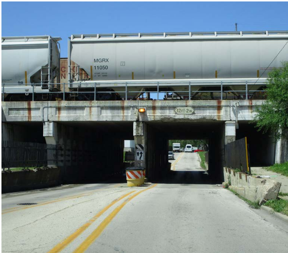
Brookmont Boulevard Viaduct in Kankakee
