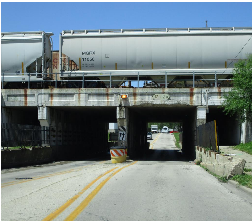
Brookmont Boulevard Viaduct in Kankakee
