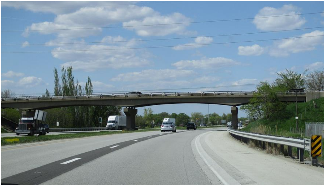
I-57 at Larry Power (4000N) Road
