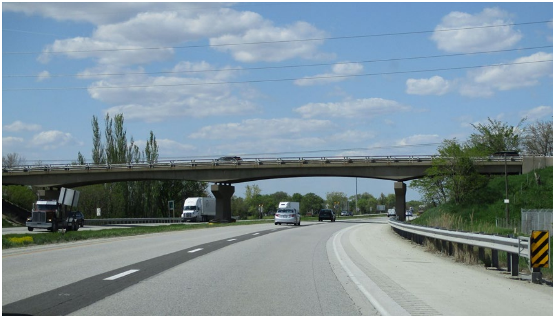
I-57 at Larry Power (4000N) Road
