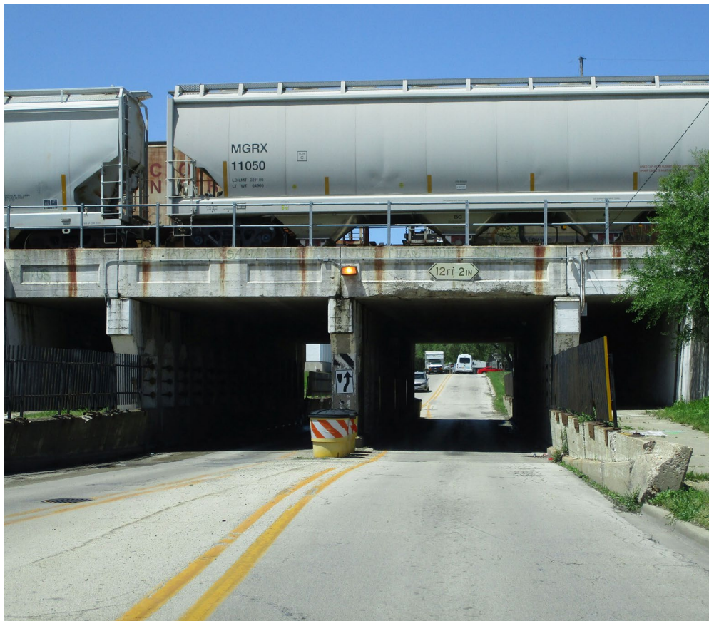
Brookmont Boulevard Viaduct in Kankakee
