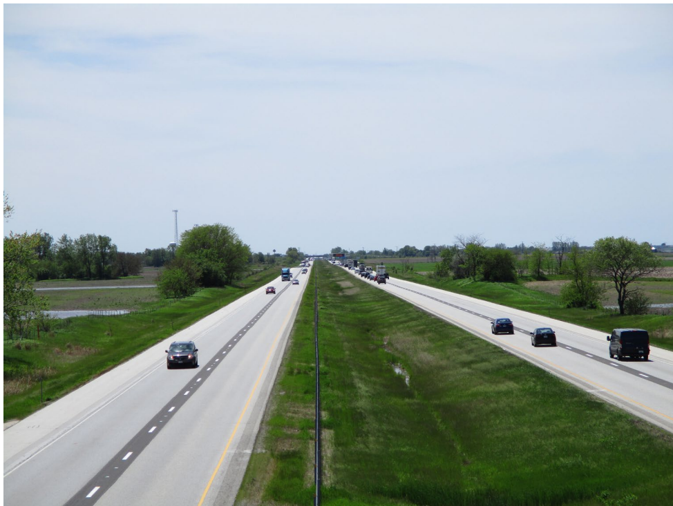
I-57 Looking South from 12000N Rd
