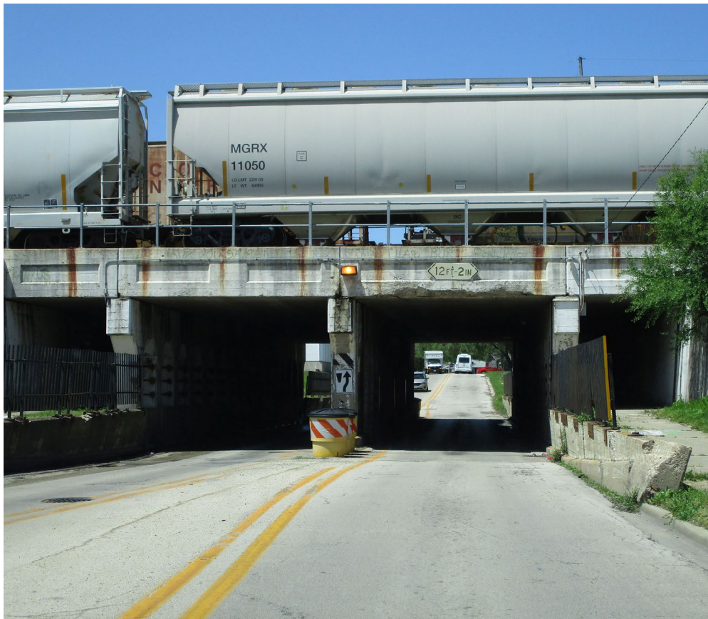
Brookmont Boulevard Viaduct in Kankakee
