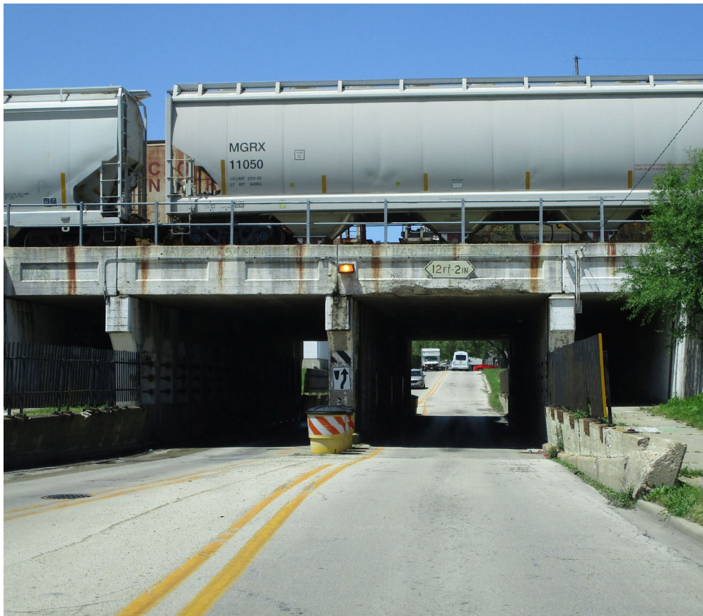
Brookmont Boulevard Viaduct in Kankakee
