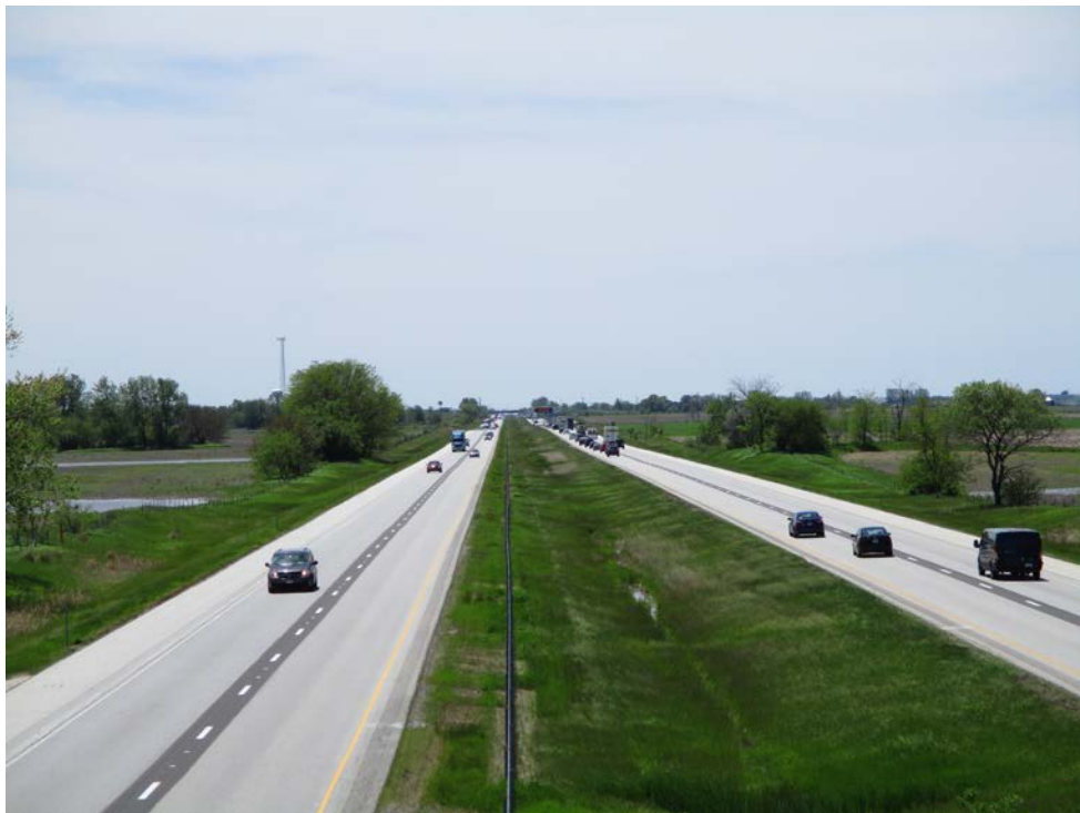
I-57 Looking South from 12000N Rd
