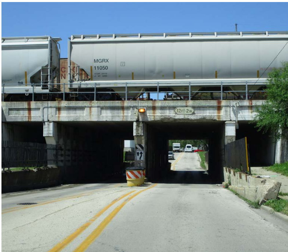
Brookmont Boulevard Viaduct in Kankakee
