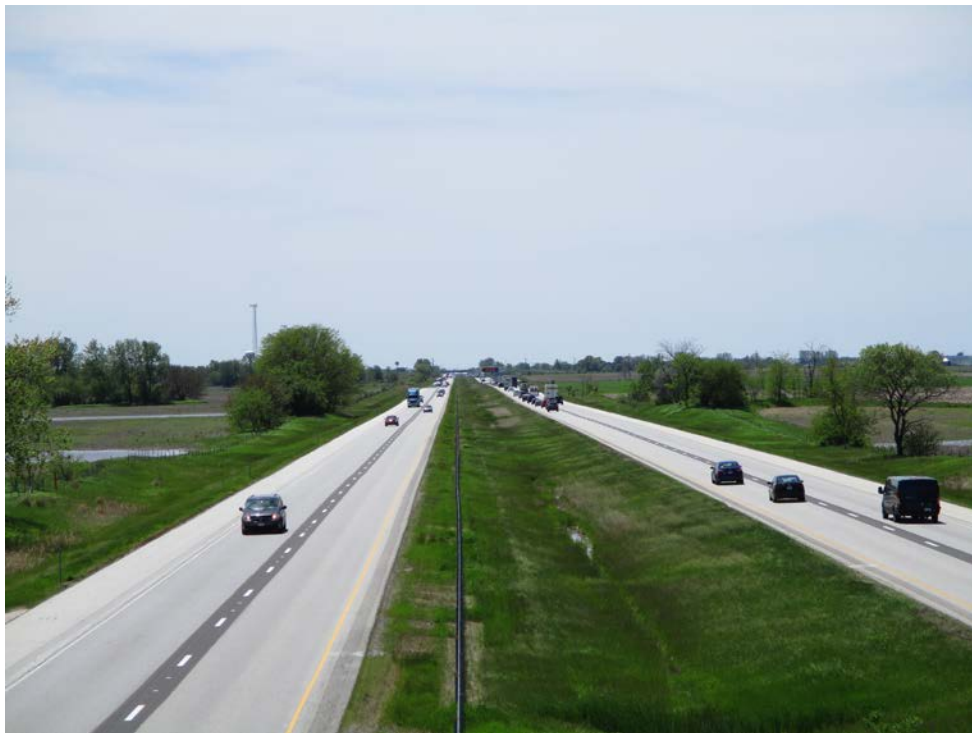
I-57 Looking South from 12000N Rd
