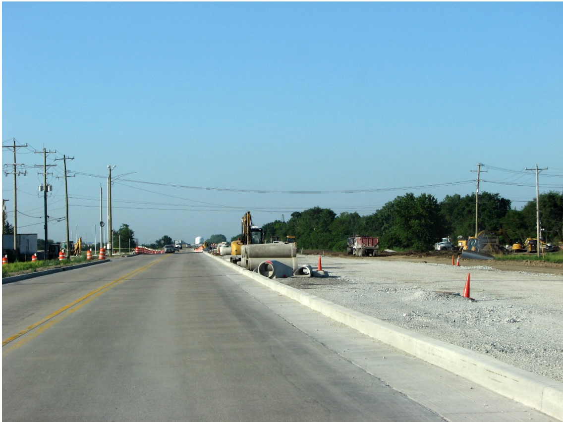
IL-50 Reconstruction at 6000N Road (June 2018)
