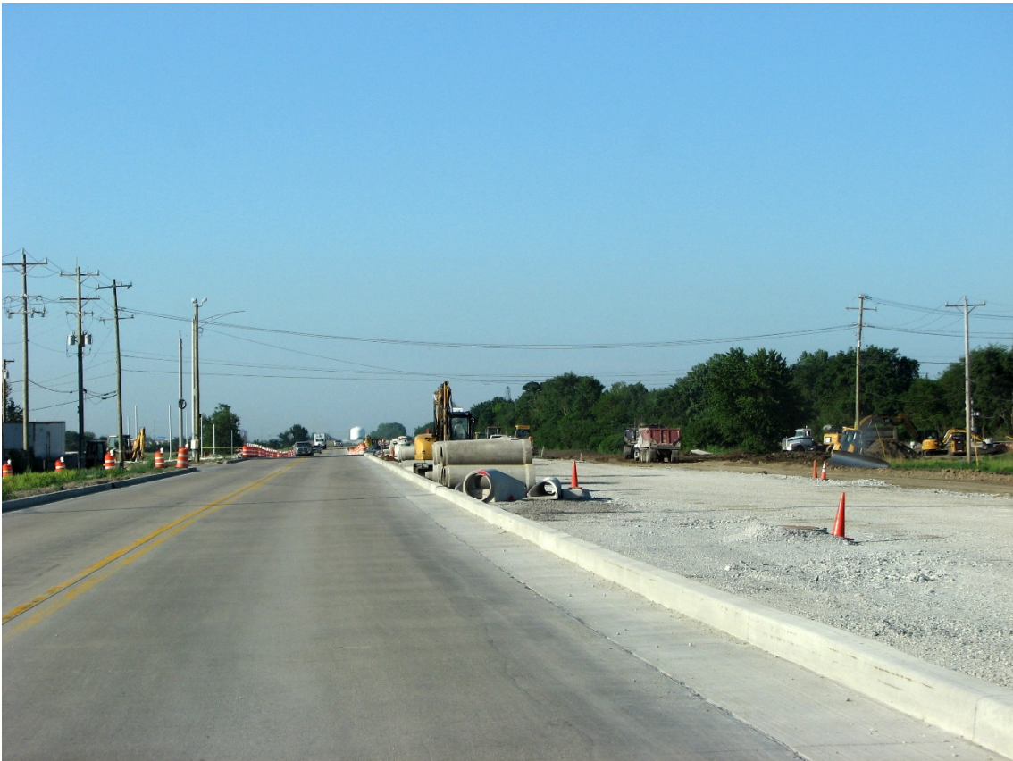
IL-50 Reconstruction at 6000N Road (June 2018)
