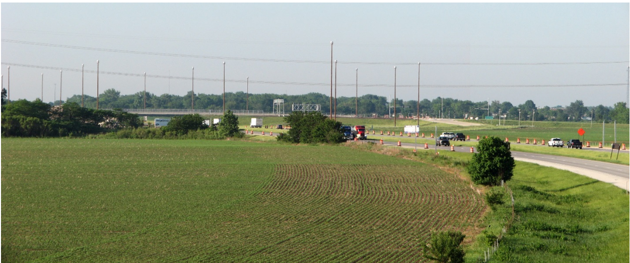
New I-57 Interchange at 6000N Road (June 2018)
