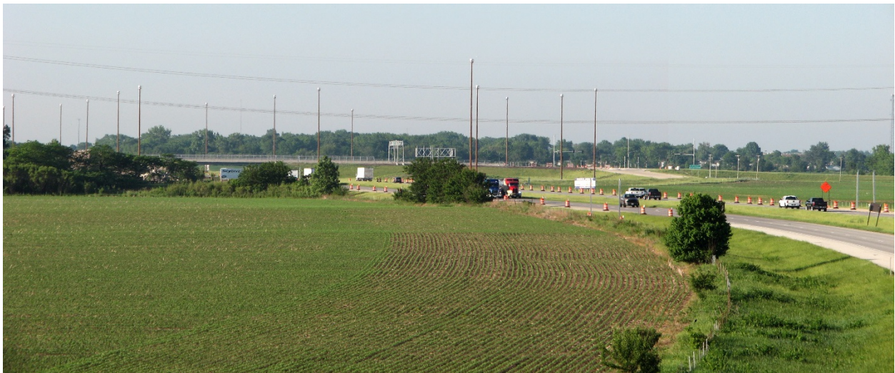
New I-57 Interchange at 6000N Road (June 2018)
