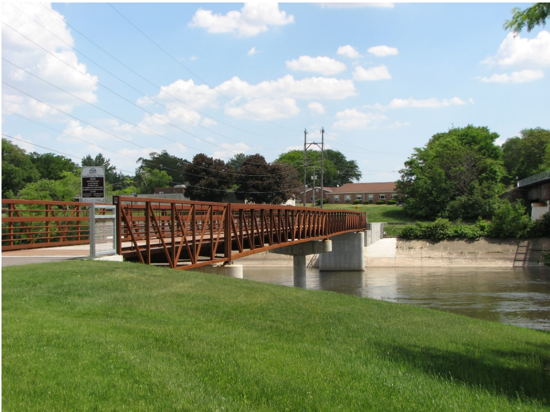
New bicycle and pedestrian bridge over the Kankakee River (May 2018)
