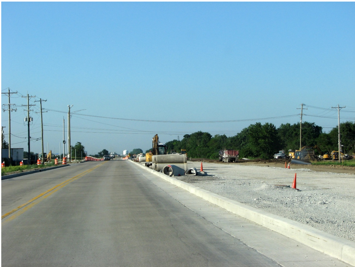
IL-50 Reconstruction at 6000N Road (June 2018)
