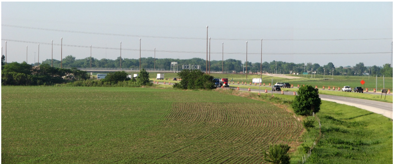
New I-57 Interchange at 6000N Road (June 2018)
