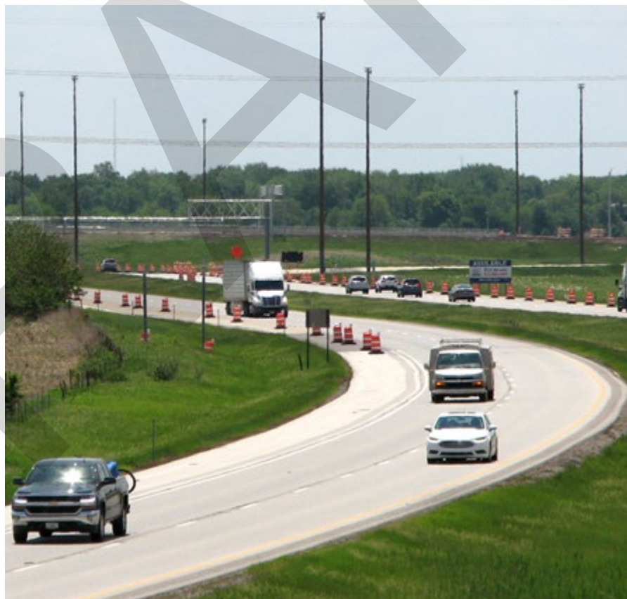
Traffic on Interstate 57 during the reconstruction of Bourbonnais Parkway.
