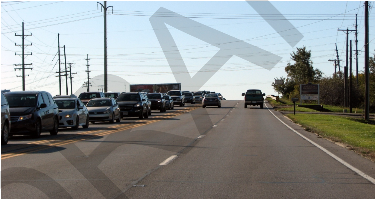
Eastbound traffic on Armour Road, west of Arthur Burch Dr., backed up to the bridge over the Canadian National (ICG) Railroad.
