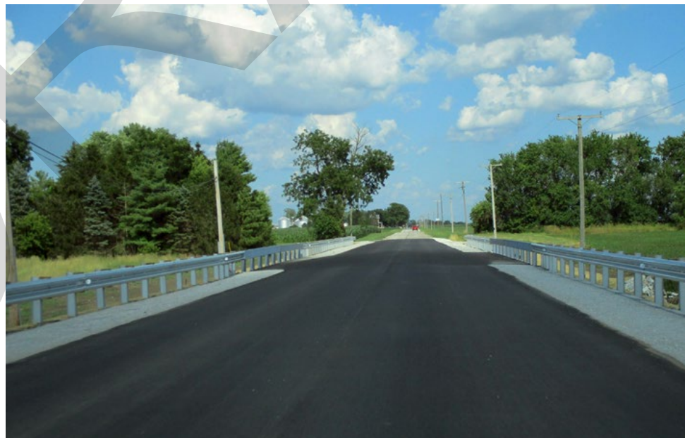
4000N Road over Solder Creek.
