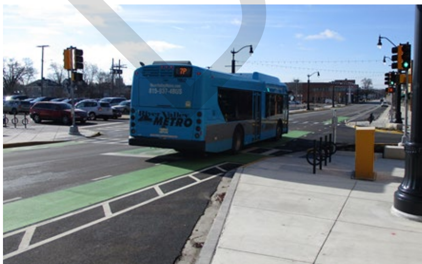
New bike lanes along Schuyler Avenue in Kankakee.
