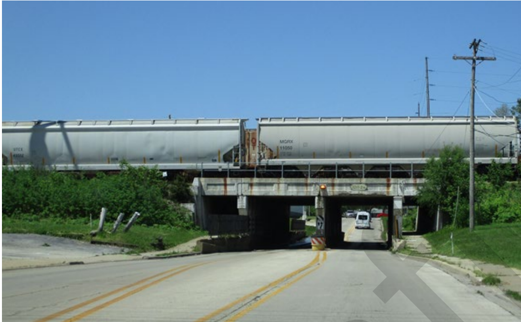
Brookmont Boulevard Viaduct (10) is a Tier 1 project.
