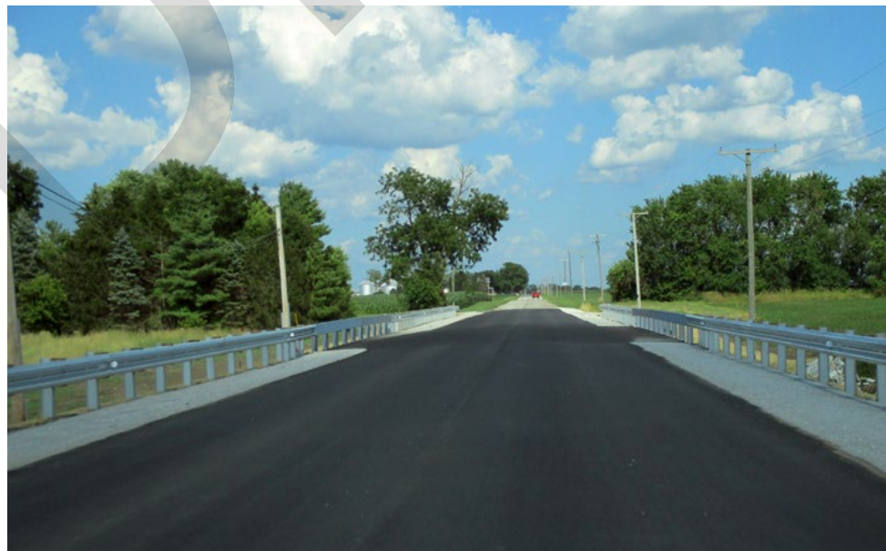
4000N Road over Solder Creek.
