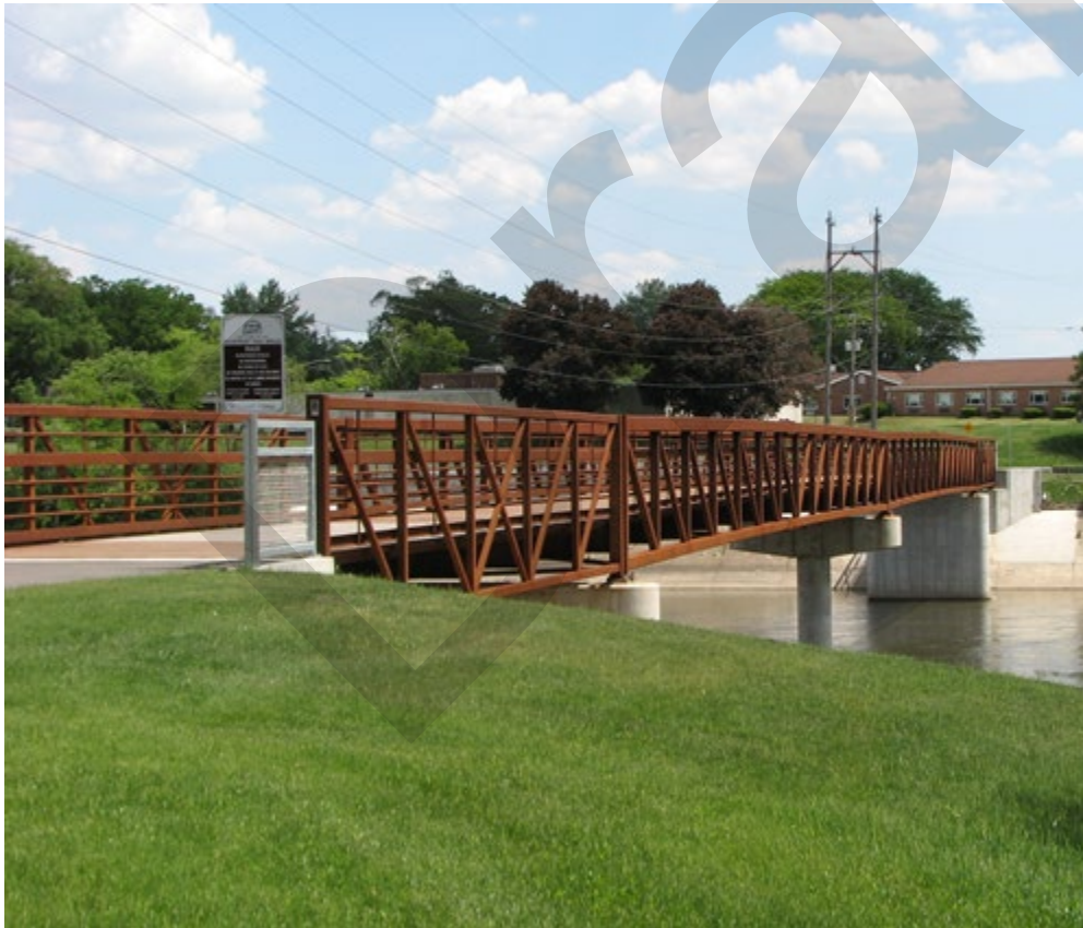
The Kankakee Riverfront Trail Bridge was completed in 2017.
