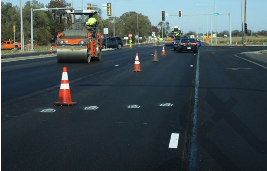
Milling and Resurfacing at the junction of Illinois State Routes 1 and 17.
