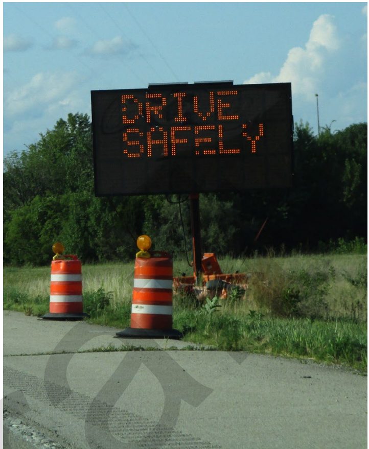
Dynamic message signs are a common form of ITS infrastructure.
